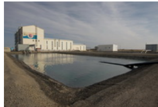
Akbastau Site Facilities
