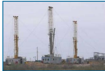
Well field development at Kharasan
