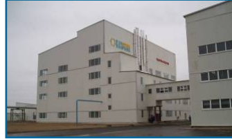
Kharasan processing facilities
