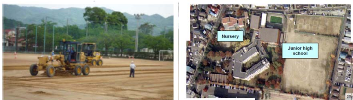
Figure 12: Example of demonstration of decontamination of school yard
