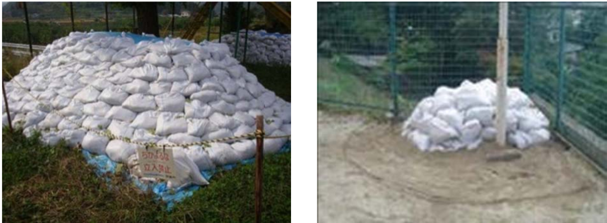
Figure 13: Temporary storage of contaminated material – examples from clean-up demonstration tests
